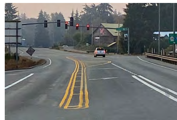
After: Traffic and striping conditions
