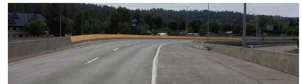
After: 2-foot tall, wide yellow band on the face of the barrier within Curve 2
