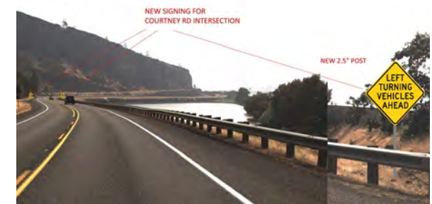
New Signage approaching Courtney Road Intersection.
