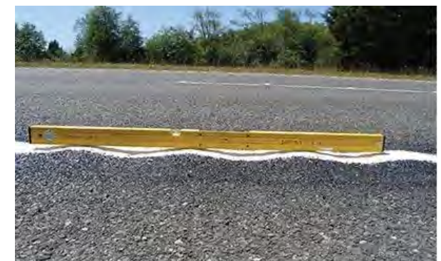
A sinusoidal mumble strip can reduce ambient noise while still alerting drivers of imminent lane departure
