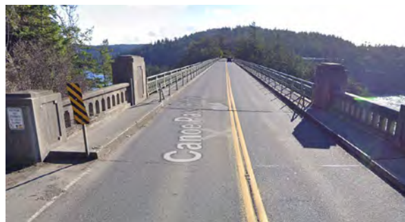
View of the bridge entrance before the project was installed.
