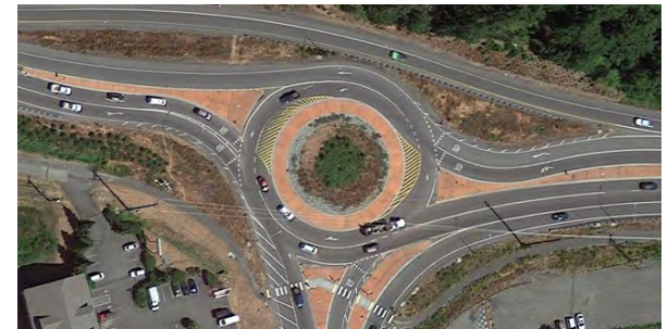
After: Southbound exit leg reduced to a single lane, with subsequent upstream channelization changes.
