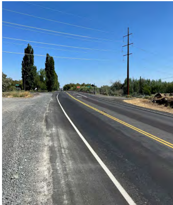
After: Minor Widening and Restriping.
