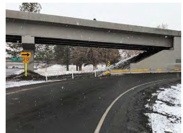
After: Upgraded signage and warning devices.
