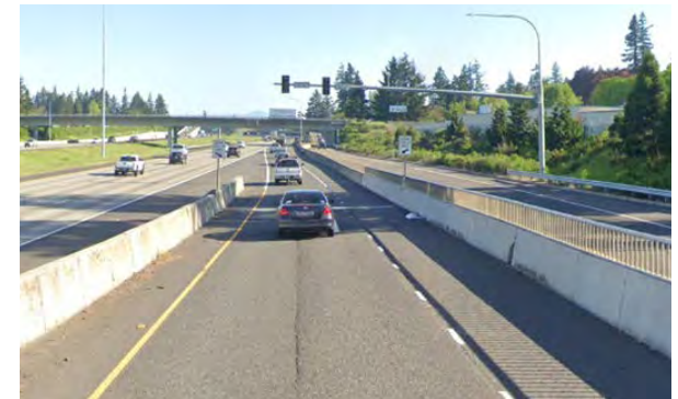
After Meter Installation.
