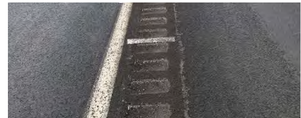
After: New rumble strips and proposed paint line.
