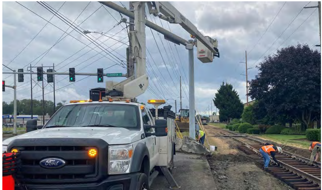
Wavetronix detection being installed on SR 432 at Industrial Way & Washington Way.
