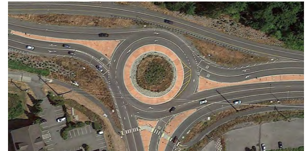
Before: Sharpes Corner roundabout with two eastbound entering lanes and two southbound exiting lanes (2x2 configuration).
