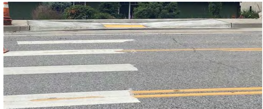
After view of the crosswalk and pedestrian ramp connection.
