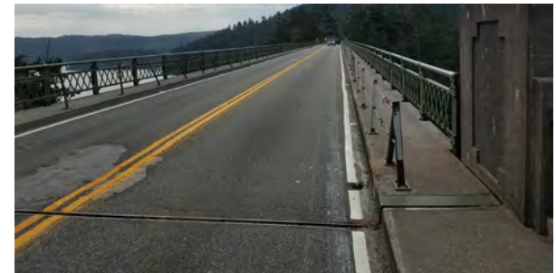
New 4" plastic edge line and reflective tape on bollards.
