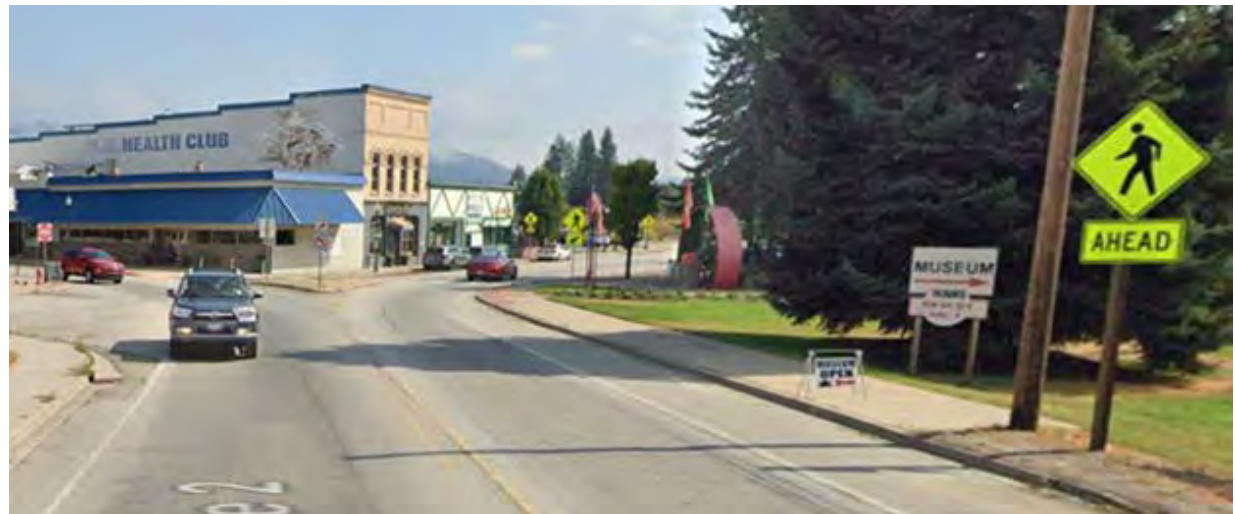
After: New pedestrian signing installed
