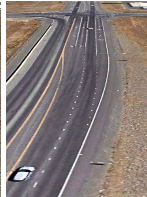
After: New lane configuration with the right lane as the thru lane and right turn pocket. The left lane ends with dual left turn lanes.
