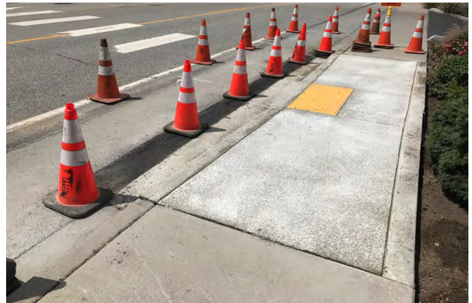
Ramp connection to pedestrian crossing during construction.
