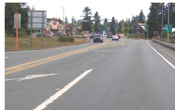
Before: Traffic and striping conditions
