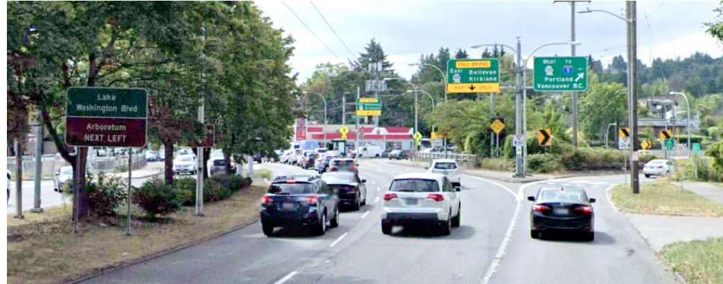
Side-mounted sign (left) and cantilever truss support system (right) on Montlake Blvd in Seattle
