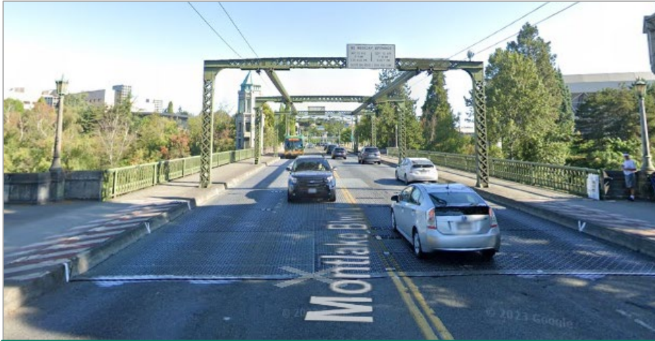
Decorative/more historic looking sign and trolley wire structure on the Montlake Bridge
