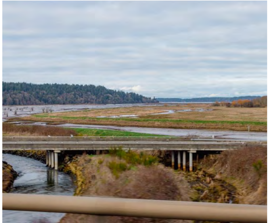
View from I-5 southbound, looking northwest
