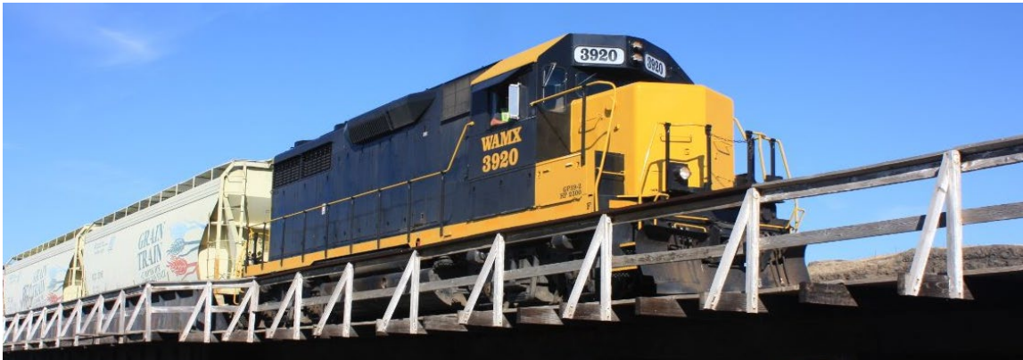
Figure 6: Picture of Grain Train on Rail Bridge
