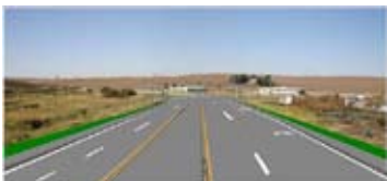
SR 270 - Pullman to Idaho State Line. WSDOT plans to widen SR 270 from two lanes to four with a 14-foot wide median lane.
