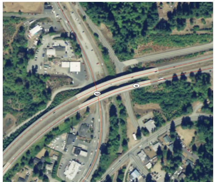
SR 169/SR 18 overcrossing with low connectivity
