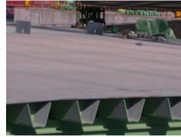
Closed Trapezoid Orthotropic Deck
