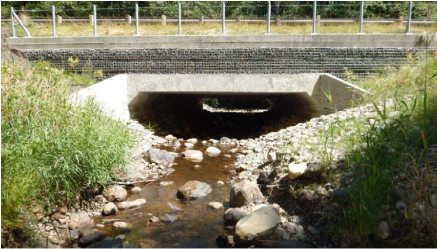
Stream simulation culvert
