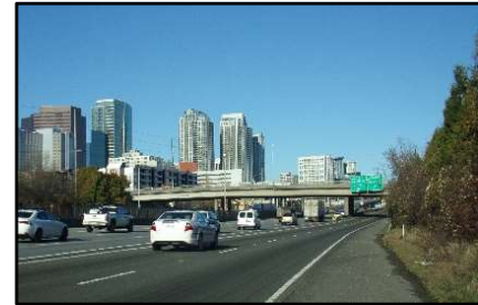
Existing Main Street Overpass
