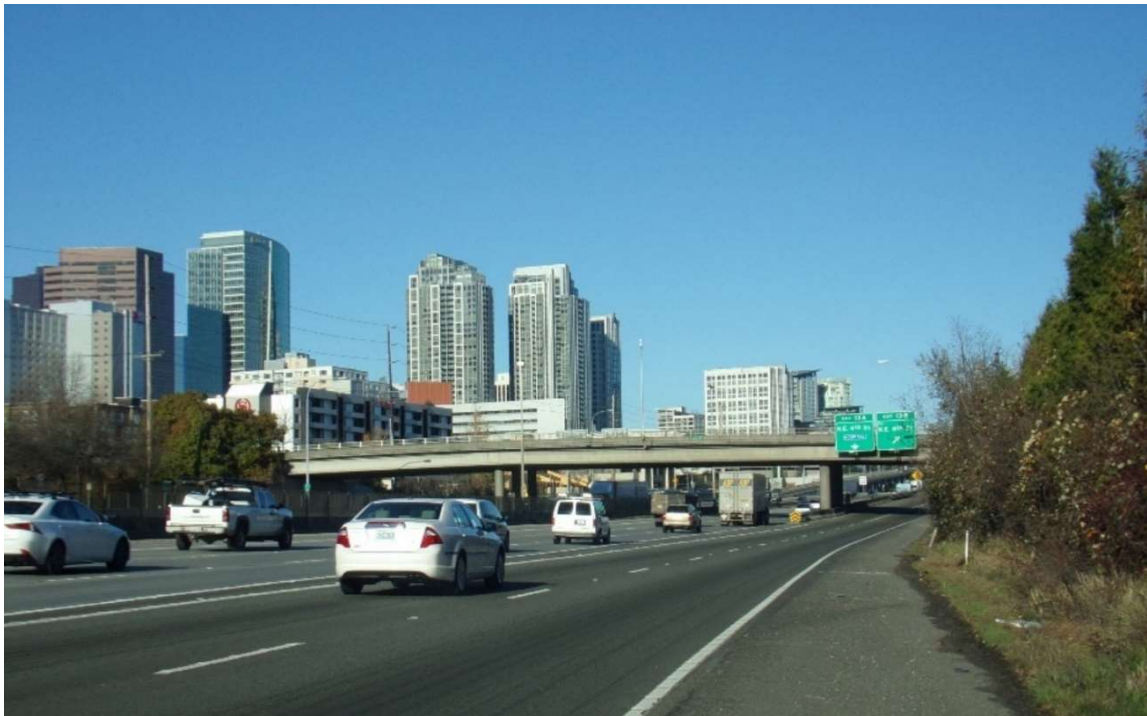
Exhibit 5-8. View C, Main Street Bridge Existing Conditions
