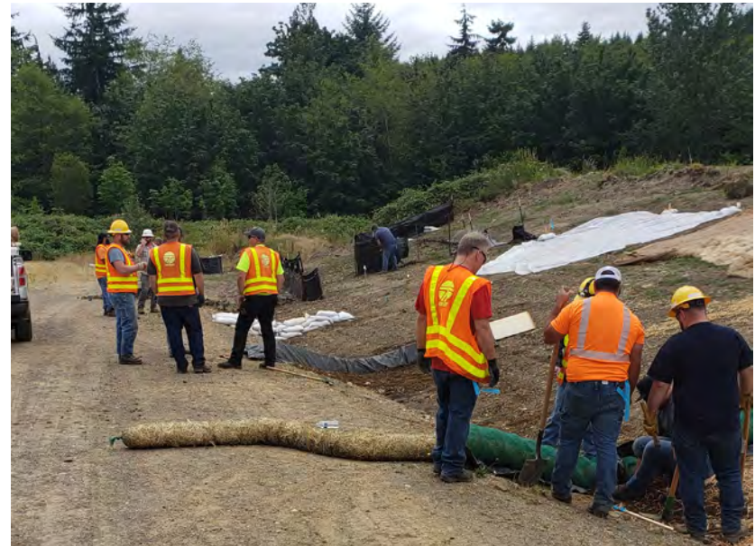
Figure 4. Participants from WSDOT's field BMP training install a check dam.
