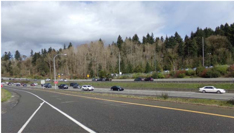
View looking northeast across I-405 near the Newport Hills Park-and-Ride lot at 112th Avenue SE
