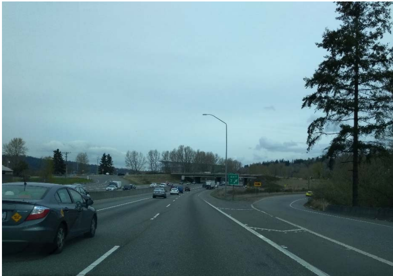
View looking north from northbound I-405 toward the NE 44th Street interchange
