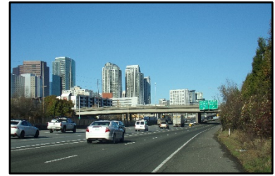
Existing Main Street Overpass
