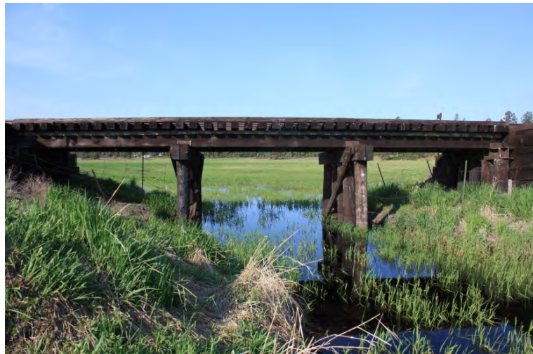
Figure 3.7: Typical Timber Trestle Bridge on P&L Branch
