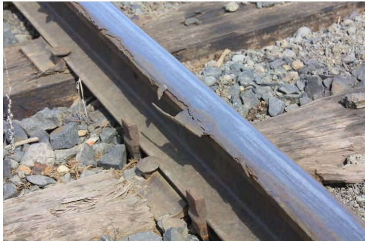
Figure 3.2: Rail Deterioration
