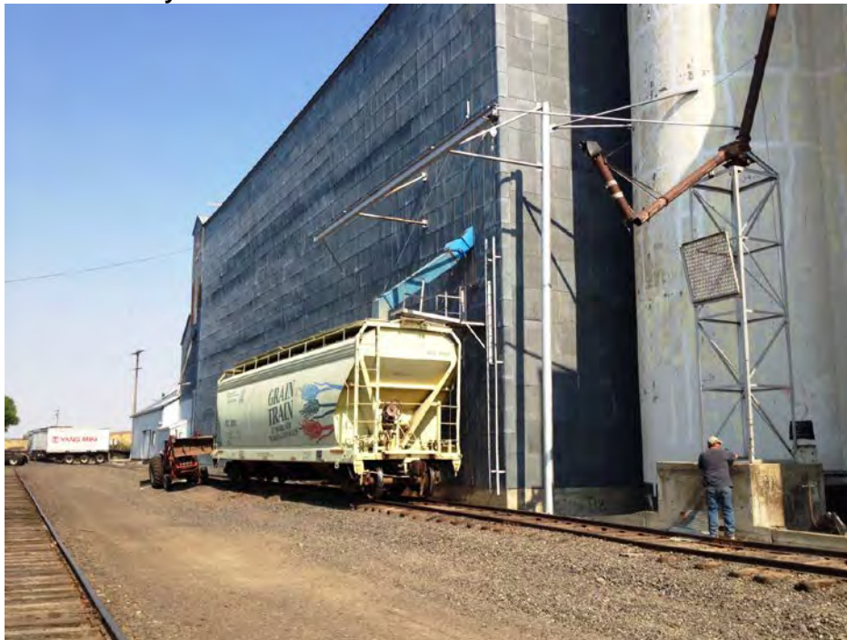
Figure 4.1: WhitGro Facility in St. John
