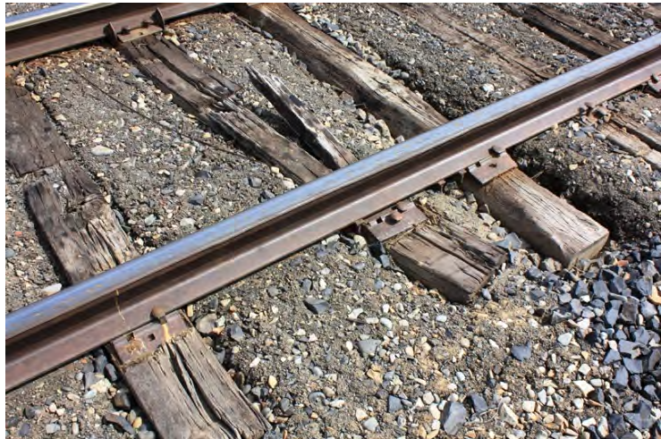
Figure 3.3: Ties on the CW Branch
