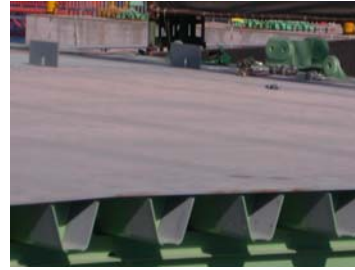
Closed Trapezoid Orthotropic Deck
