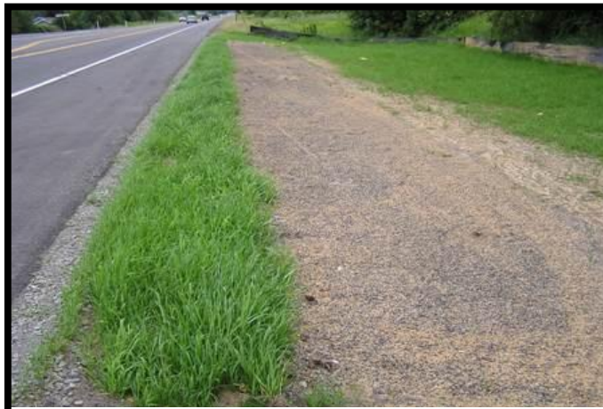
Media Filter Drain Along SR 167 in King County
