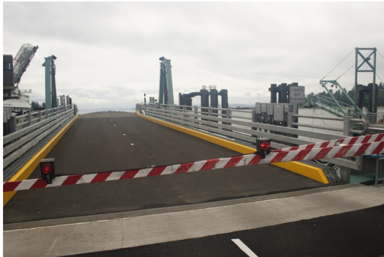
Bainbridge Island Vehicle Transfer Span (H-Span) Exhibit 610-3
