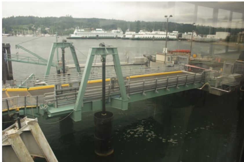
Bainbridge Island Hydraulic Transfer Span (H-Span) Exhibit 610-1
