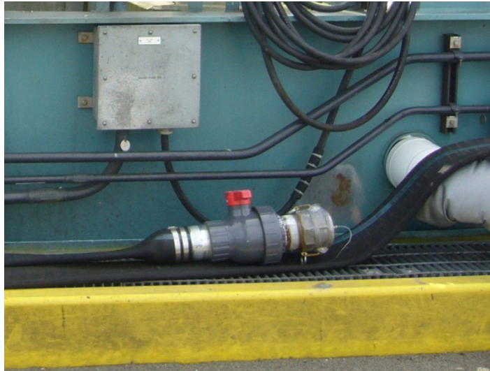
Sewer Line Connection Exhibit 610-14
