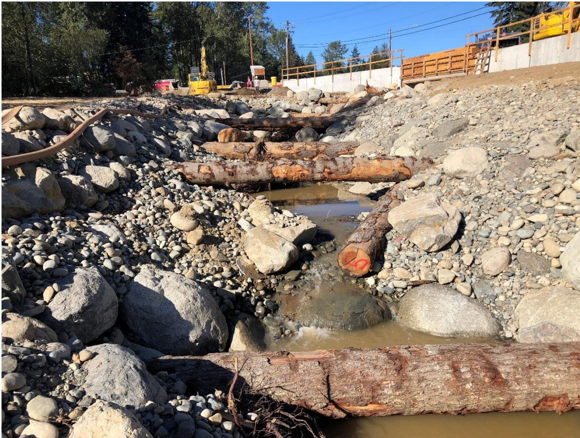
Image taken from a project in Centennial Creek, Snohomish County. This was a fish passage barrier correction.
