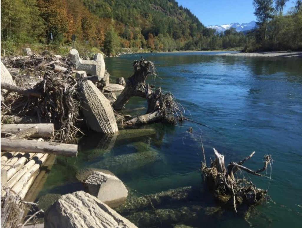
Figure 10A-9 Dolotimber Structures, Skagit River, Skagit County
