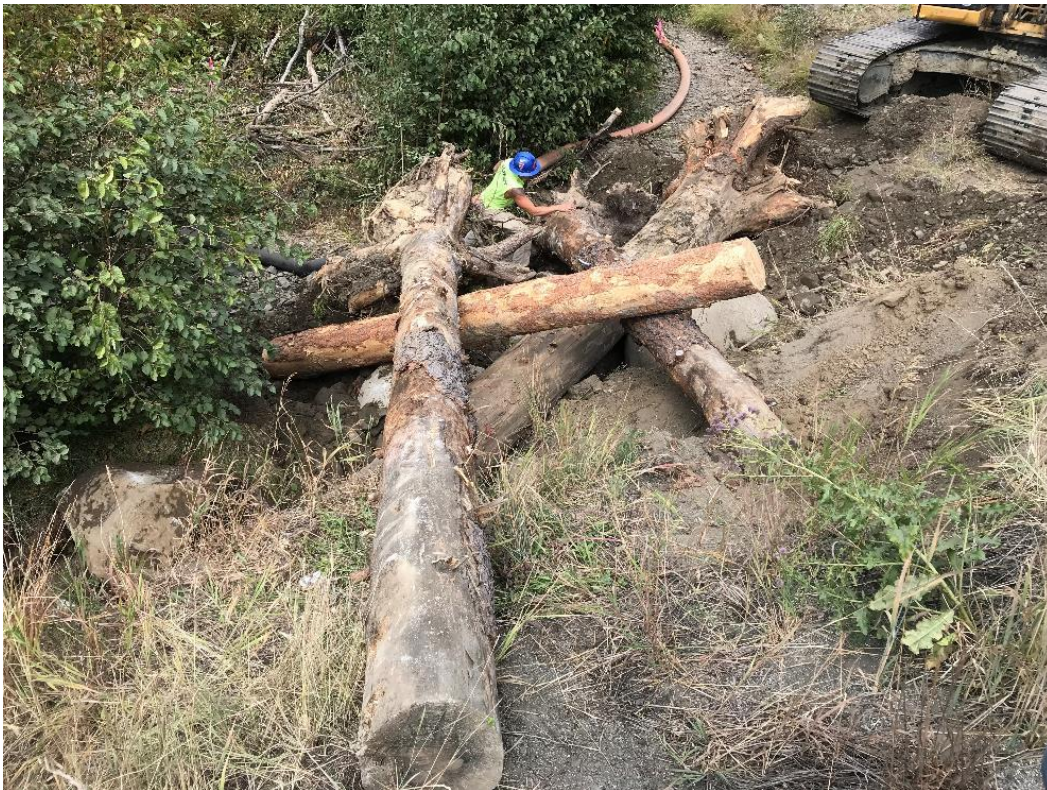
Figure 10A-1 Self-ballasting Large Wood Structure, Swauk Creek, Kittitas County
