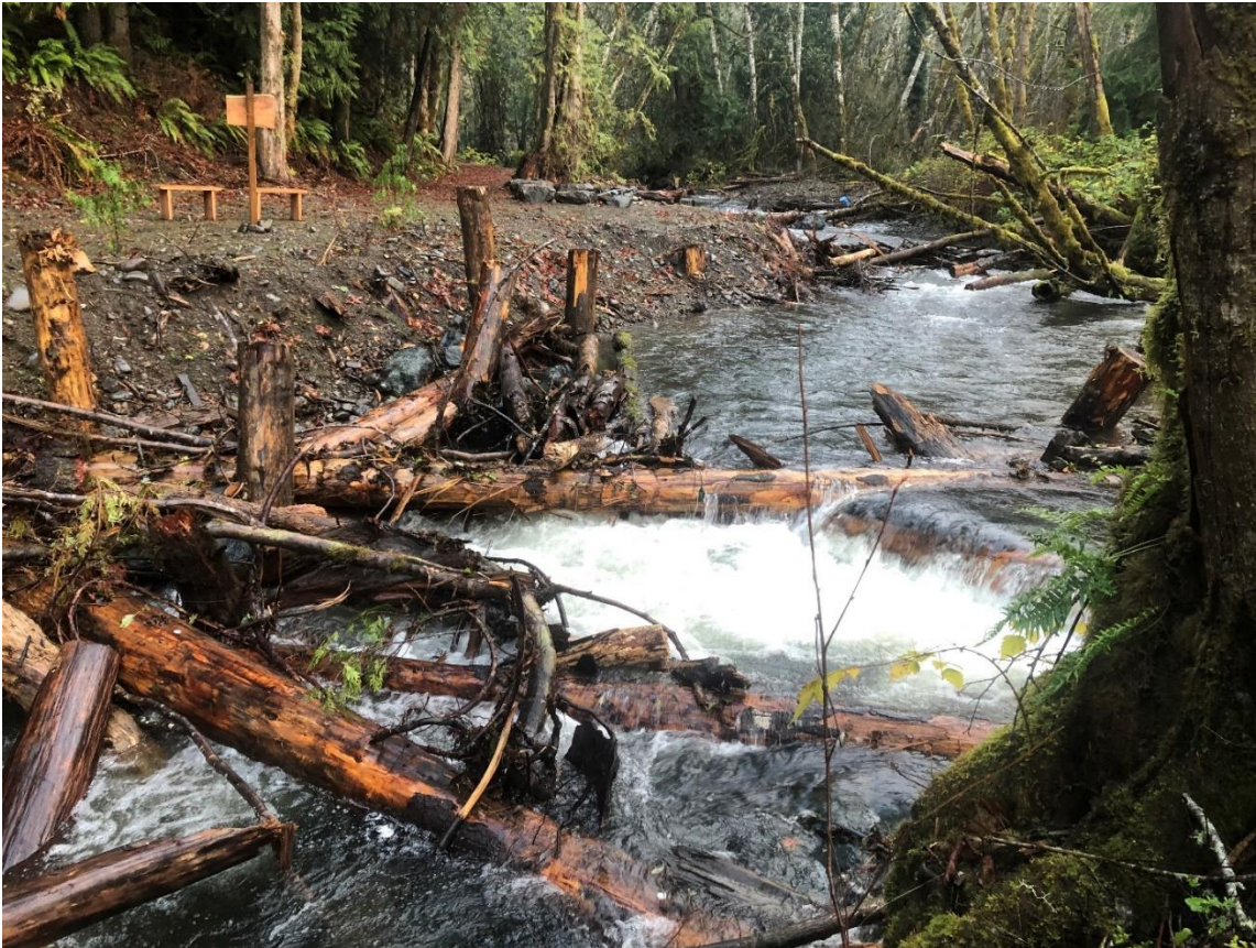
Figure 10-6 Example of Small-Channel Complex Log Grade Control
