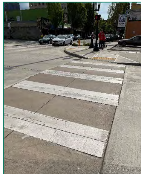
FIGURE 58. ADA CURB RAMP IN OLYMPIA, WA.
