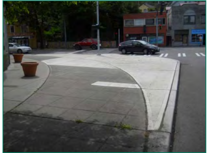
FIGURE 20. TIGHTER CURB RADIUS. SOURCE: PEDSAFE.
