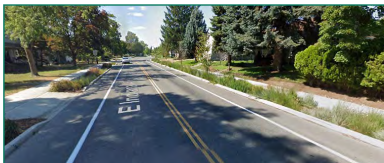
FIGURE 2. EAST INDIANA AVENUE ROAD RECONFIGURATION IN SPOKANE, WA. SOURCE: GOOGLE MAPS.
