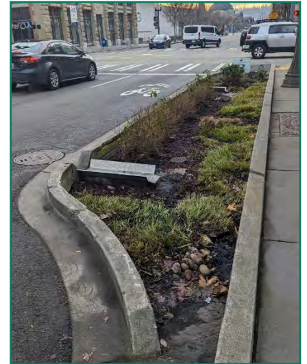
FIGURE 23. PHYSICAL BARRIER TO RESTRICT PARKING IN TACOMA, WA. SOURCE: DONGHO CHANG.
