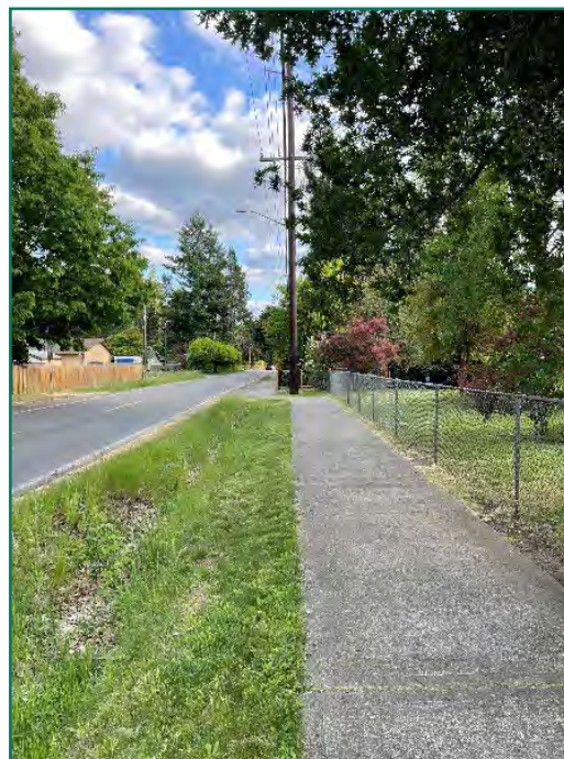
FIGURE 68. SEPARATED WALKWAY WITH BIOSWALE IN OLYMPIA, WA.
