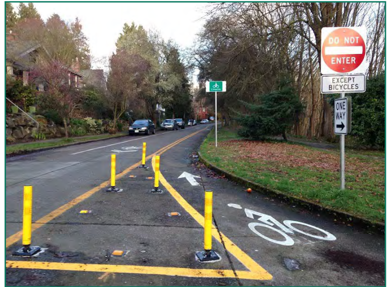
FIGURE 64. CONTRAFLOW BIKE LANE IN SEATTLE, WA. SOURCE: DONGHO CHANG.
