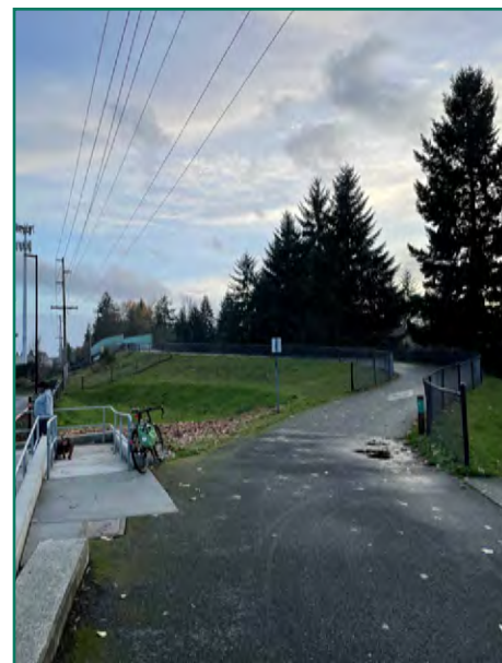
FIGURE 53. PEDESTRIAN/BICYCLIST OVERPASS IN OLYMPIA, WA.
