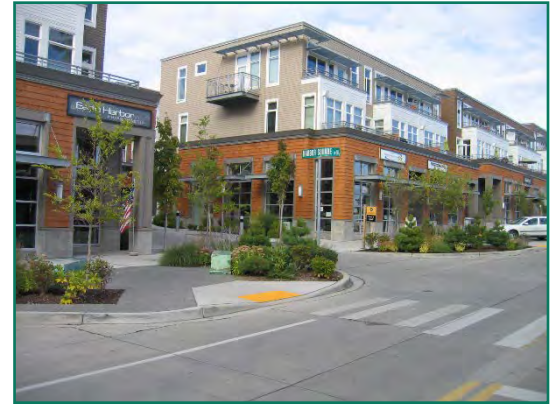
FIGURE 24. CURB EXTENSION ON BAINBRIDGE ISLAND, WA. SOURCE: PEDBIKE IMAGES/CARL SUNDSTROM.
