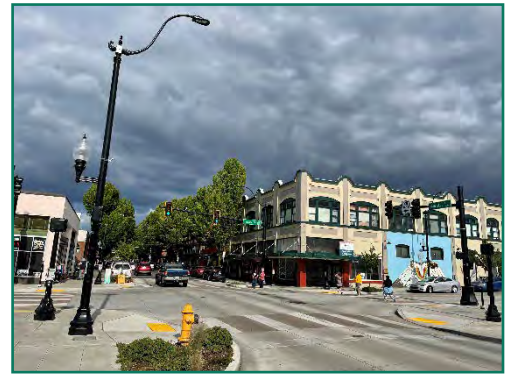
FIGURE 42. TRAFFIC SIGNAL IN OLYMPIA, WA
