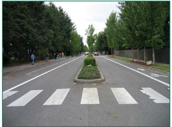
FIGURE 27. HIGH-VISIBILITY CROSSWALK IN UNIVERSITY PLACE, WA. SOURCE: PEDBIKE IMAGES/CARL SUNDSTROM.
