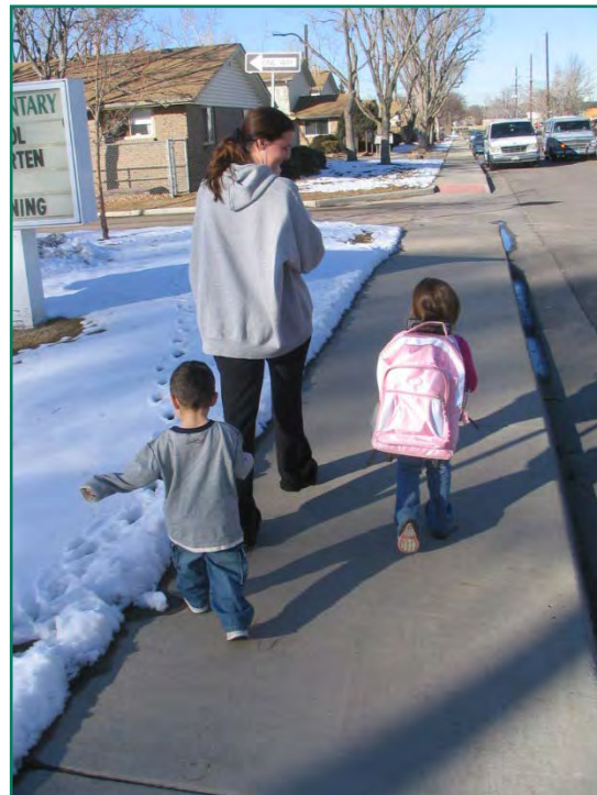
FIGURE 66. SIDEWALK WITHOUT BUFFER. SOURCE: PEDBIKE IMAGES/DAN BURDEN.
