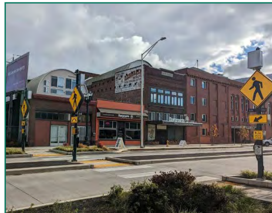
FIGURE 38. RRFB IN EVERETT, WA. SOURCE: DONGHO CHANG.
