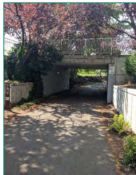
FIGURE 54. PEDESTRIAN/BICYCLIST UNDERPASS IN SPOKANE, WA.
