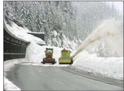
Avalanches in the project area regularly close I-90.
