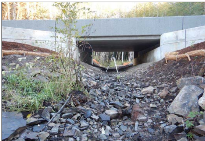
Figure 41. Outlet of the Wooster Creek crossing immediately after construction, October 2018.
