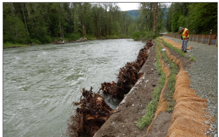
Figure 8. Sauk River Side Channel post-construction, May 2020.
