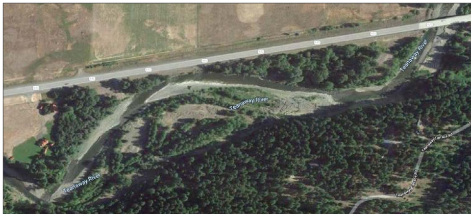
Figure 16. SR 970 Teanaway River CED project vicinity. The river has been encroaching on SR 970 since 1991, which has resulted in erosion and flooding of the roadway multiple times over the years. A CED project is scheduled for construction in 2022.
