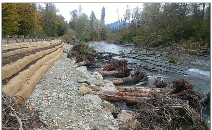
Figure 5. Sauk Side Channel interim maintenance repair, September 2019.
