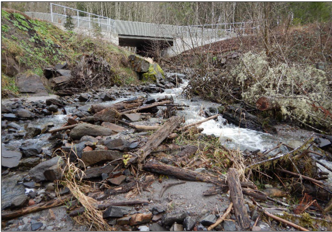
Figure 44. Downstream of Wooster Cr crossing 1.5 years after construction, February 2020.
