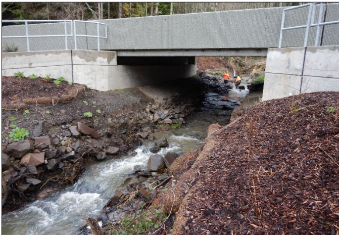
Figure 43. Channel regrade under the Wooster Cr Bridge, February 2020.
