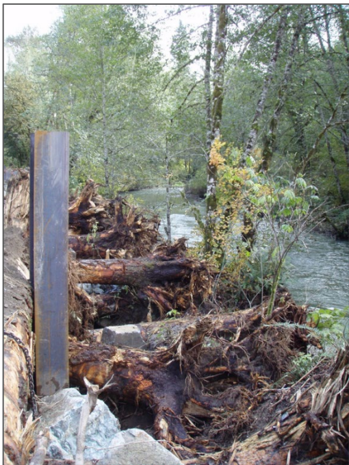
Figure 4. Sauk River Side Channel log cribwall, 2008.
