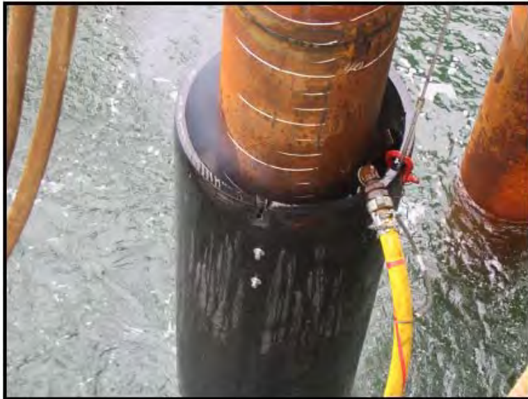
Figure F.5. Type II Confined Bubble Curtain Sleeve Deployed During Driving a Plumb Pile
