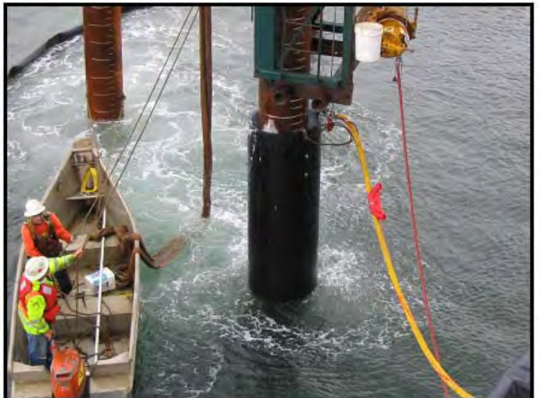
Figure F.5. Type II Confined Bubble Curtain Sleeve Deployed During Driving a Plumb Pile
