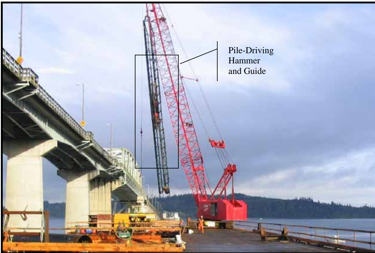
Figure 4. Impact Pile-Driving Hammer Used to Drive Monitored Piles
