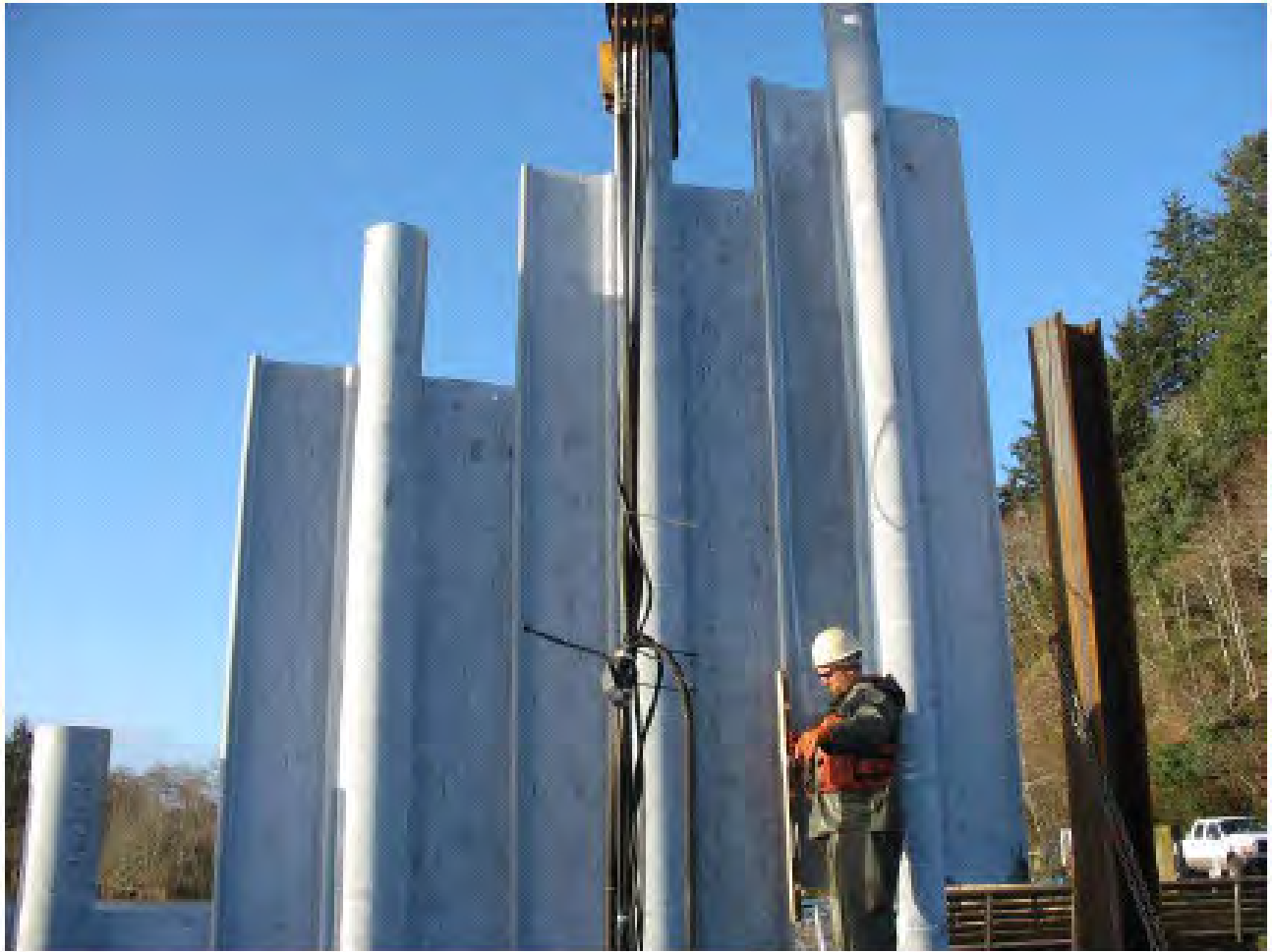
Figure 2: 12-inch diameter steel piles with interlocking ‘wings’ used to create the wave barrier (photo courtesy of Washington State Parks and Recreation, R. Johnson).
