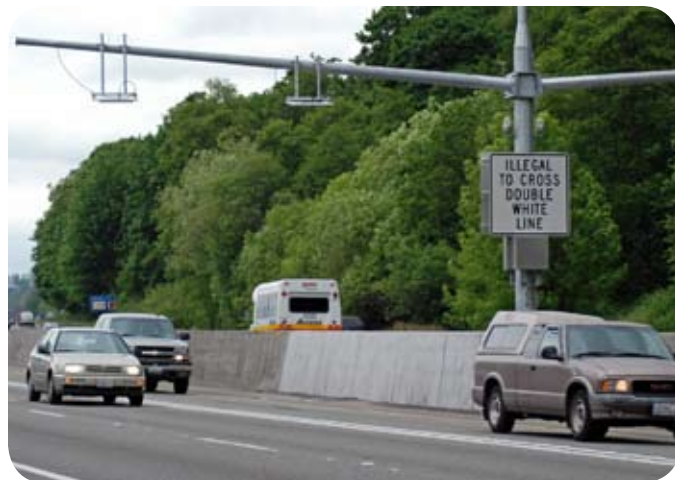
The readers for electronic tolling on SR 167 HOT lanes
