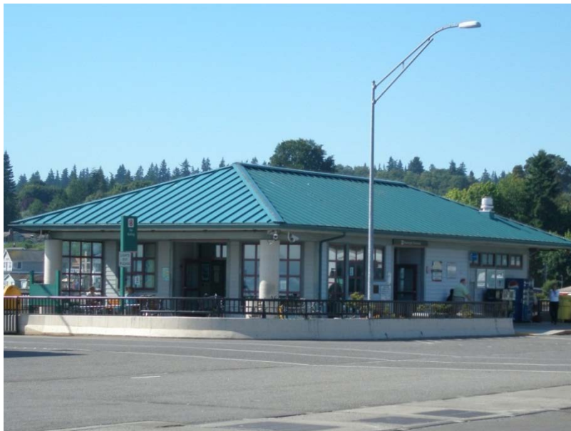
Clinton Ferry Terminal Passenger Building Exhibit 400-1
