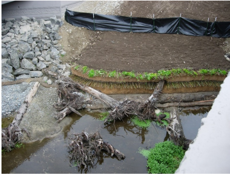
Exhibit 9: SR 18 stream restoration – use of woody material, coir lifts, and planting for bank protection.
