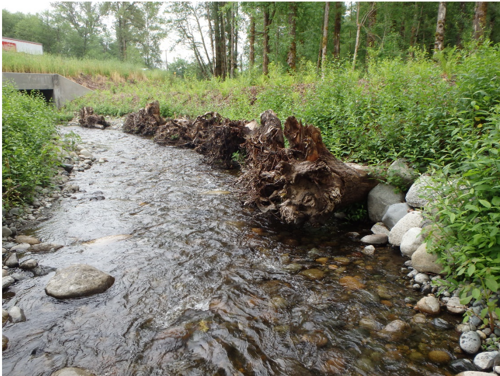
Exhibit 8: Logs and rocks used in restoration.
