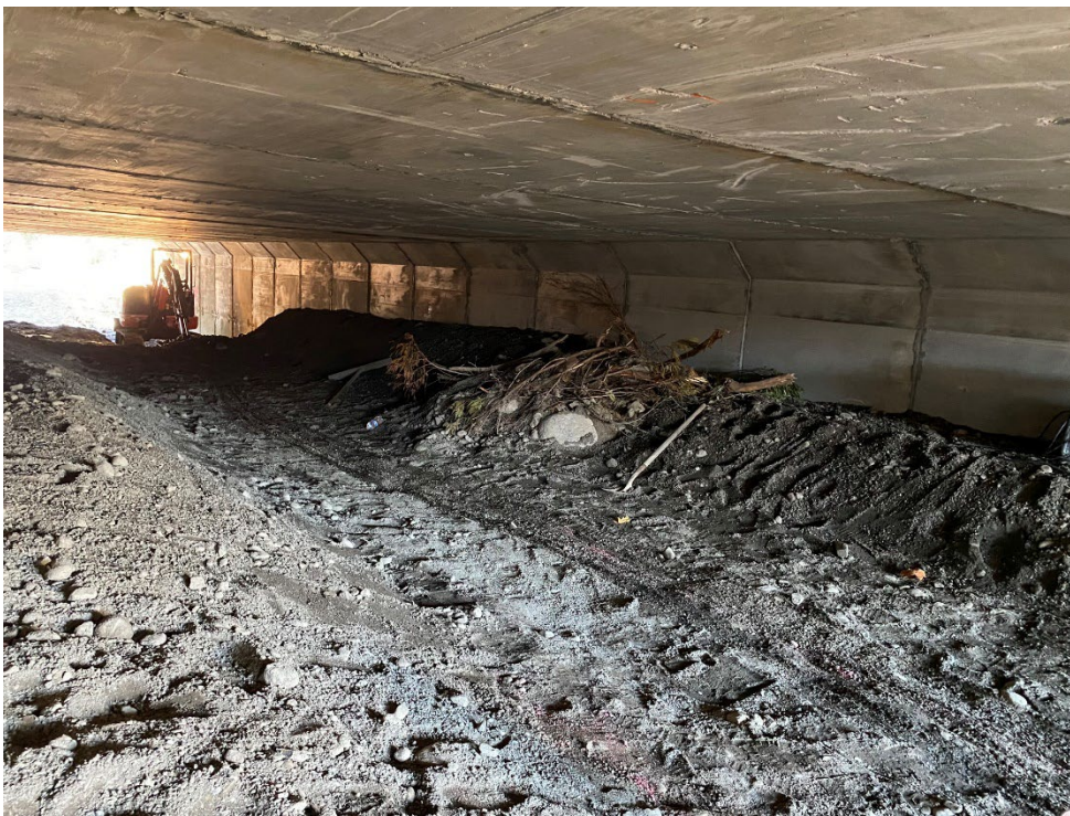
Figure 7-17 Example of a Constructed Meander Bar with Slash
