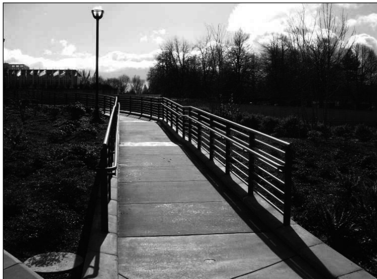
Pedestrian Access Ramp
