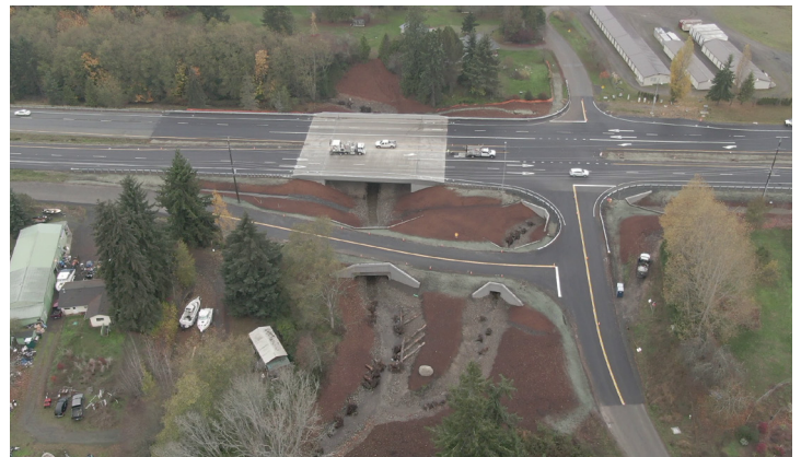
ABOVE: Bagley Creek Culvert Fish Passage
