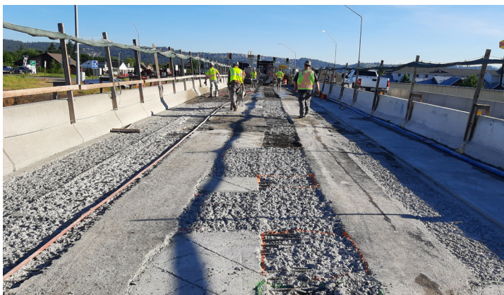
ABOVE: Mullan Bridge Deck Rehabilitation
