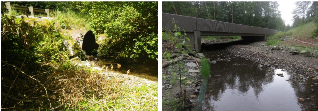
Exhibit 1: SR 9 Lake Creek. Prior to restoration, the culvert was undersized and water was restricted. Post-construction, stream is free to move through the culvert and buffers are restored with native plants.
