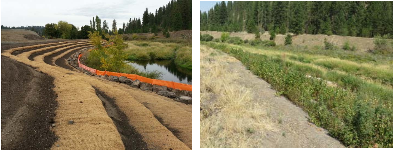
Exhibit 11: US 195 Cheney Spokane Interchange. The left photo shows coir wrapped layers prior to vegetation establishment. The photo on the right shows vegetation establishment after two years.
