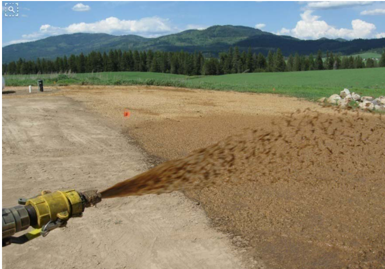
Exhibit 10: Application of hydromulch for erosion control.
