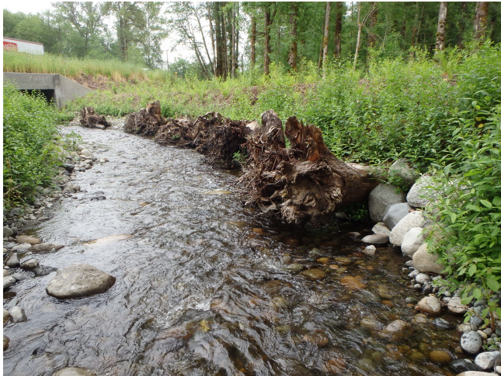
Exhibit 8: Logs and rocks used in restoration.
