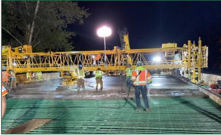
Northeast 44 th Street Interchange
