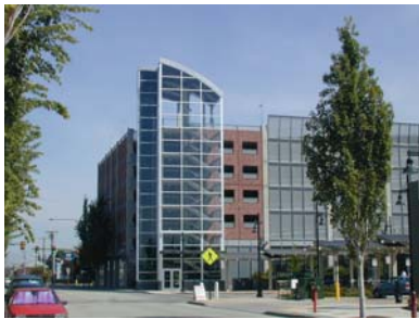
Downtown Renton Parking Garage
