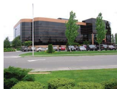
Office building in Renton's Employment Area Valley
