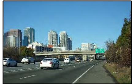
Existing Main Street Overpass
