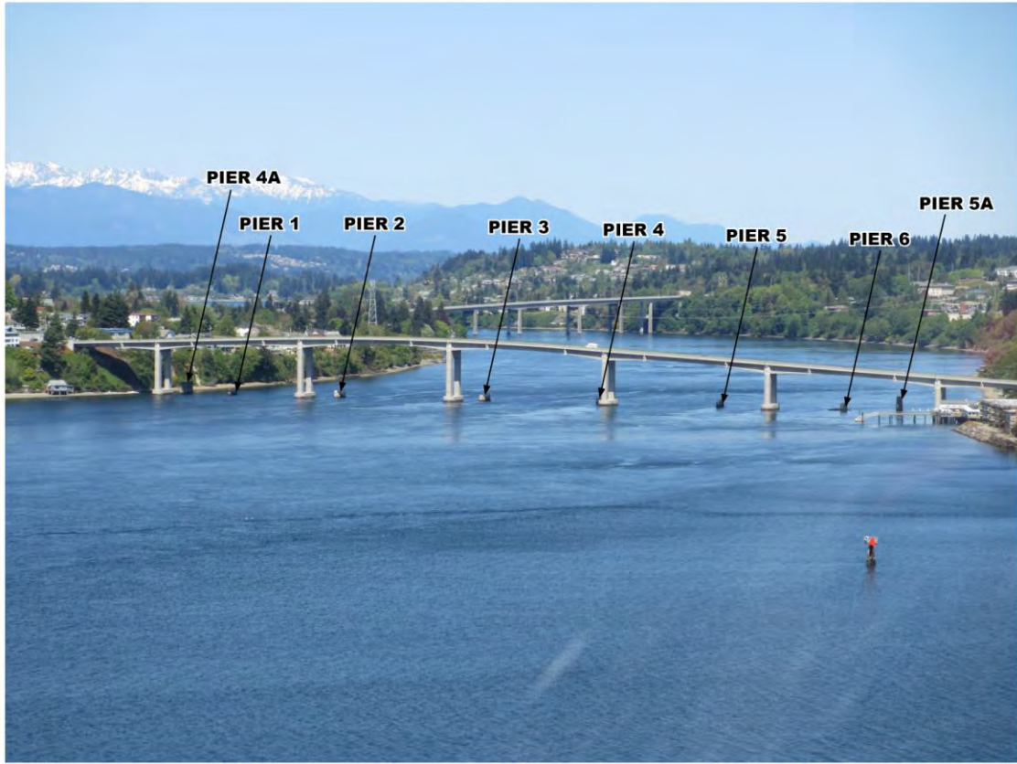
Figure 2: Location of the old concrete piers relative to the new Manette Bridge.
