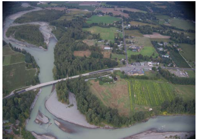
SR 542 Nooksack River Bridge to Nugent's Corner
