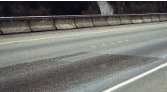
Chip Seal Repair Low
