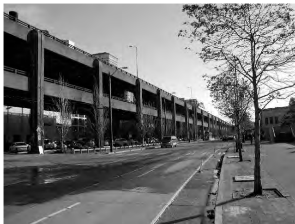
Alaskan Way Viaduct at Alaskan Way surface street and Union Street.
