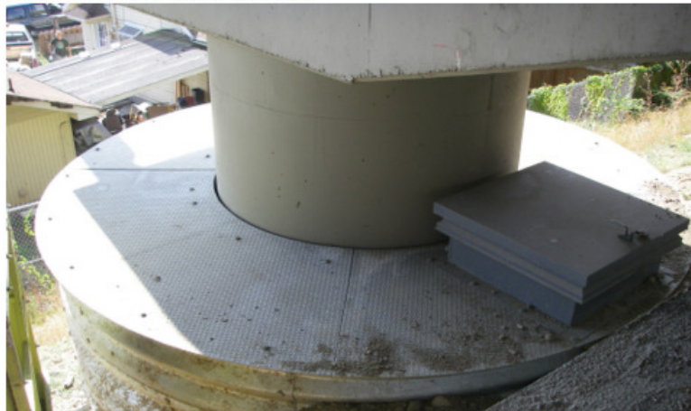
I-5 N-N RAMP OVER I-5 - 5/628N.N - 0016991A
