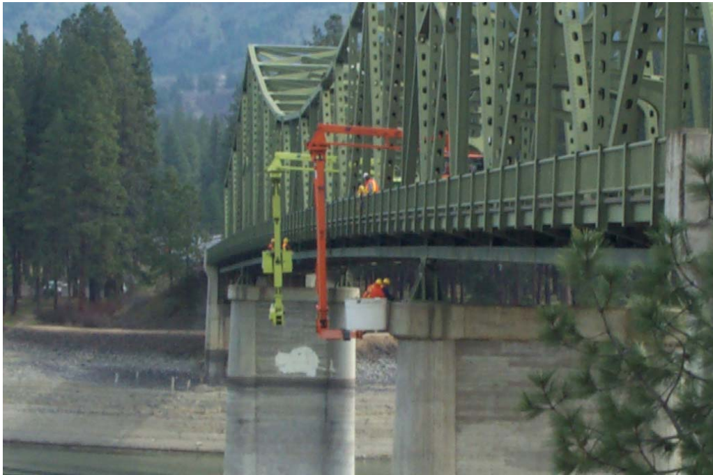
Figure 1 Typical multi-crew UBIT inspection
