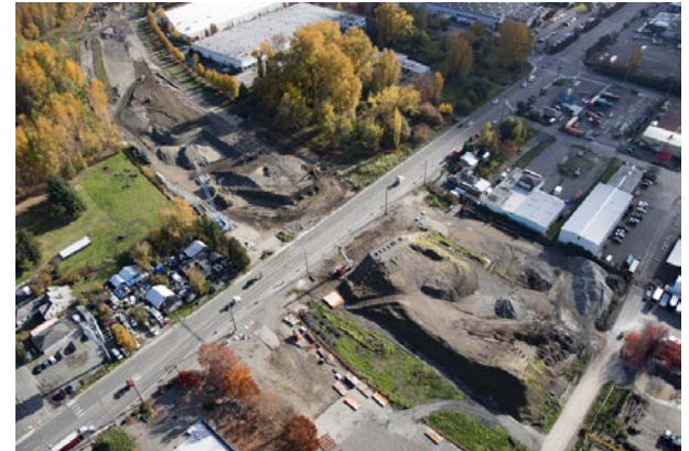
Building embankment for the new 54th Avenue interchange
