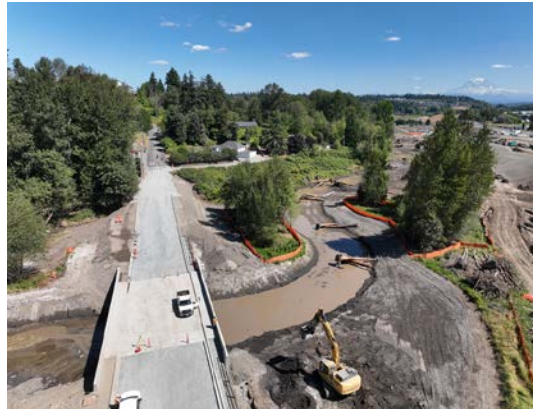
Completed 12th Street East bridge over the re-aligned Hylebos Creek
