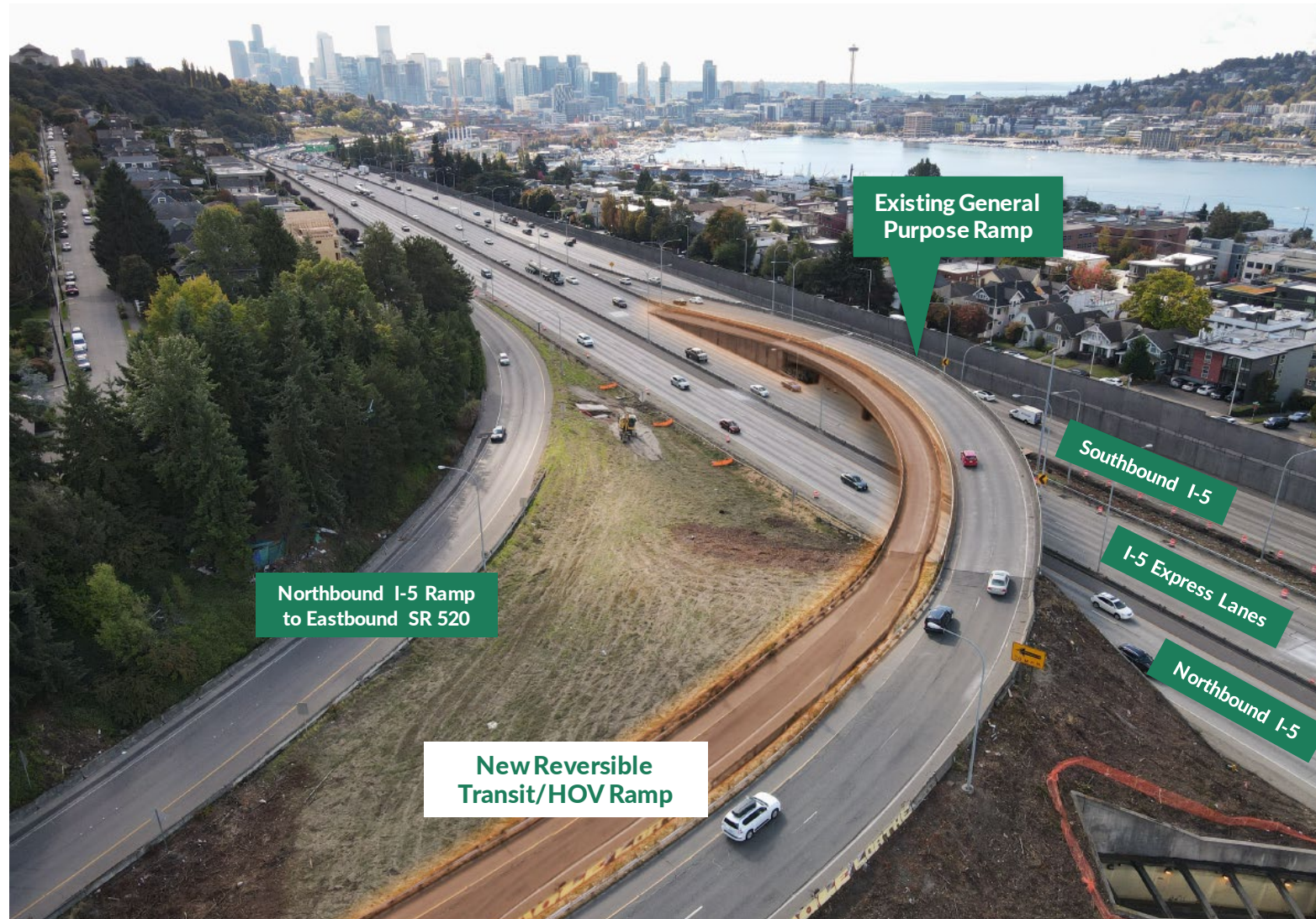
Looking south at I-5 and SR 520 interchange
