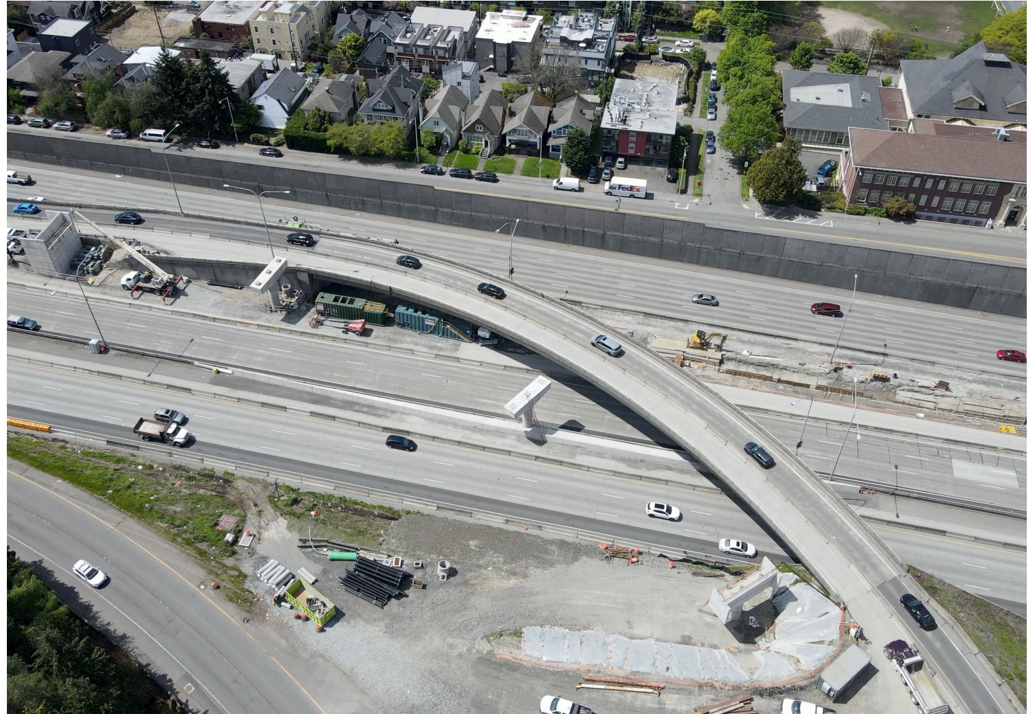
From above where the new flyover ramp will be built next to the westbound SR 520 ramp to southbound I-5.
