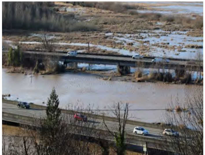
The Nisqually River delta at I-5 when the river was flowing at about 20,000 cubic feet per second and roughly 12 feet gauge height during a flood event in February 2020. This was just below a moderate-level flood event. The record flood from 1996 hit 17.13 feet of gauge height. Photo courtesy of the Nisqually Indian Tribe.
