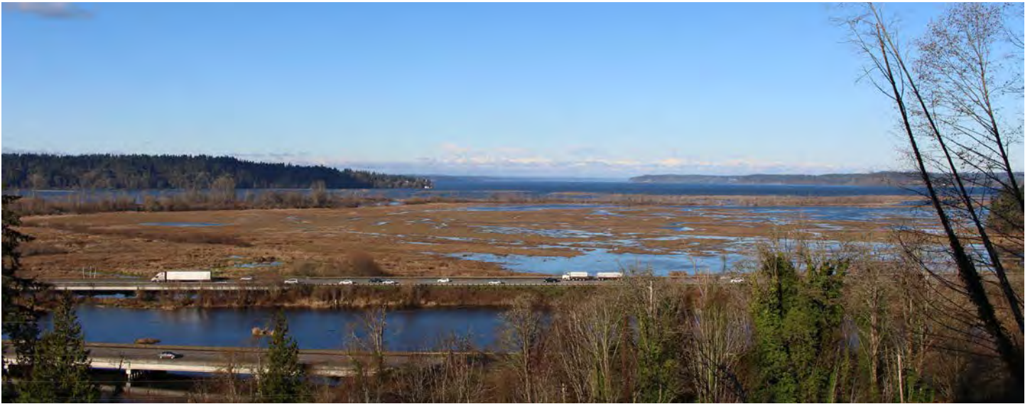
The Nisqually River delta and Interstate 5 with Puget Sound in the background. I-5 traverses through the Nisqually River valley adjacent to the delta, important habitat for Endangered Species Act-listed Chinook salmon and steelhead.
