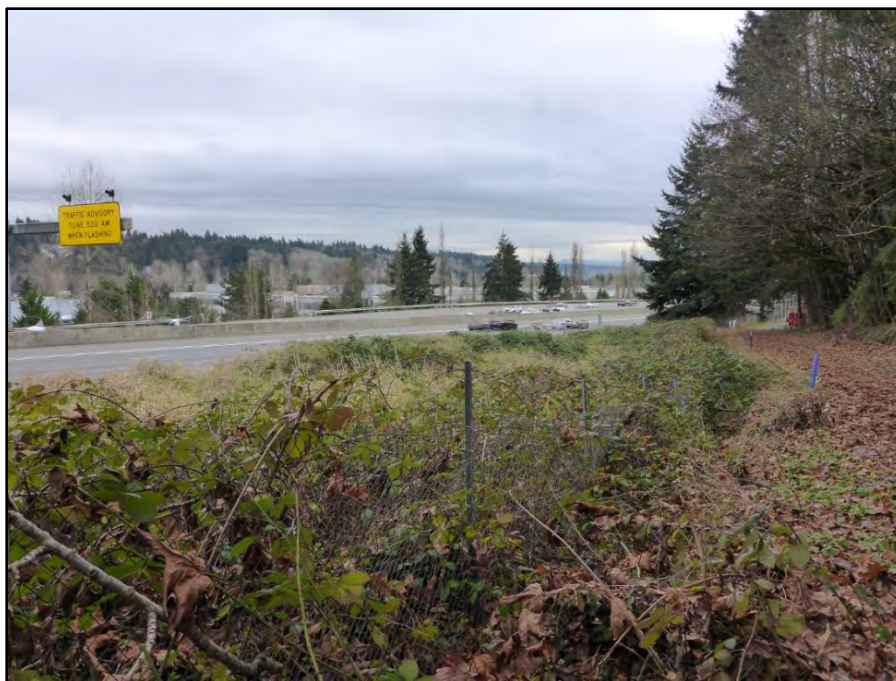
Exhibit 2. Overview of the Stream 25.0L-West study area from the north end. The existing lanes of I-405 mark the eastern boundary of the study area in this view to the southeast.
