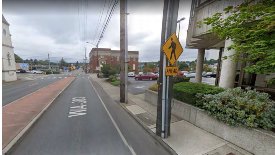
Figure 19. Existing Roadway Characteristics – Sidewalk Obstructions
