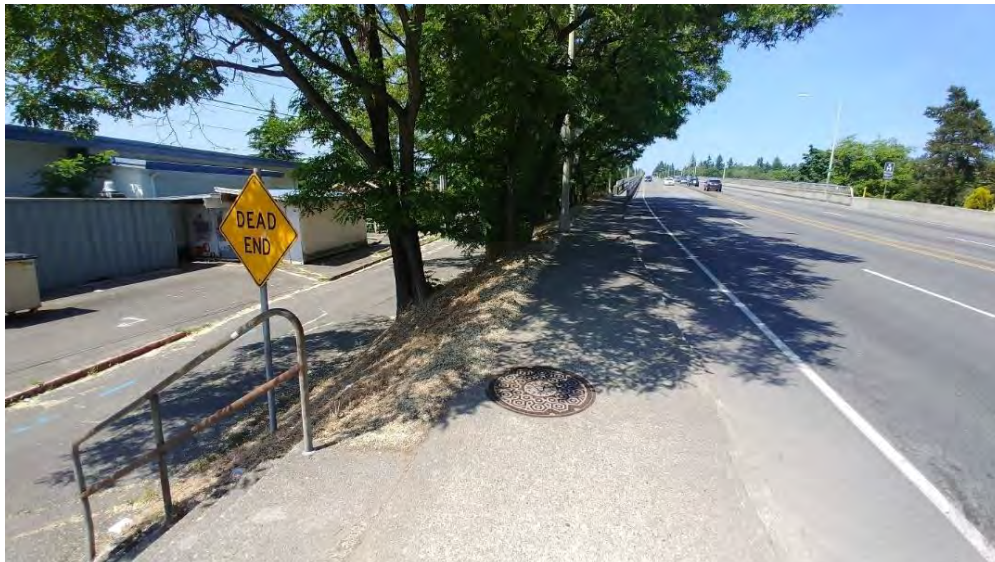
Figure 23. Existing Roadway Characteristics – Warren Avenue Bridge Sidewalks
