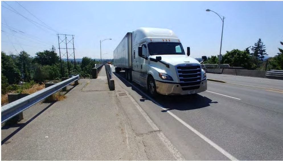
Figure 24. Existing Roadway Characteristics – Warren Avenue Bridge Sidewalks
