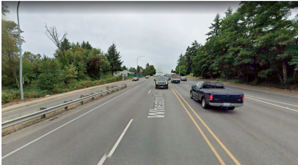
Figure 26. Existing Roadway Characteristics – Callahan Drive Sidewalk Gaps
