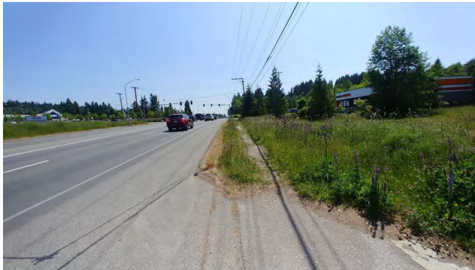
Figure 31. Existing Roadway Characteristics – Sidewalk Gaps
