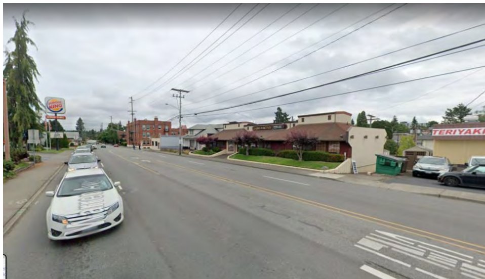
Figure 18. Existing Roadway Characteristics – 6th Street TWLTL
