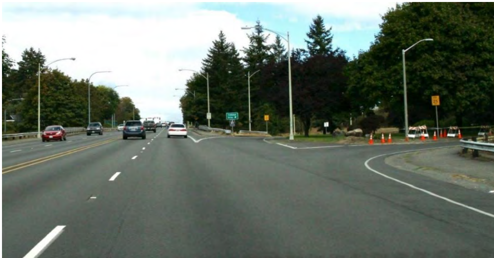
Figure 25. Existing Roadway Characteristics – Callahan Drive Ramps
