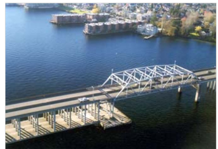
West highrise of Evergreen Point Bridge
