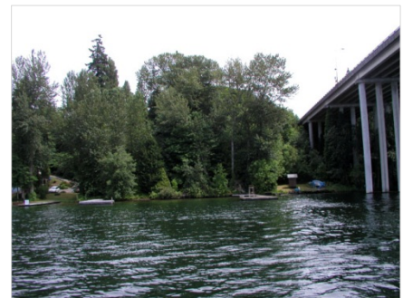
Eastern shoreline of Lake Washington north of the east approach structure
