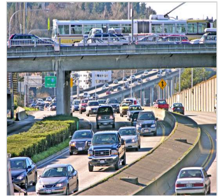
Local buses traveling over SR 520 on the Montlake Boulevard overpass
