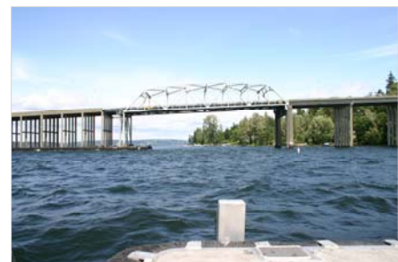
East highrise of Evergreen Point Bridge
