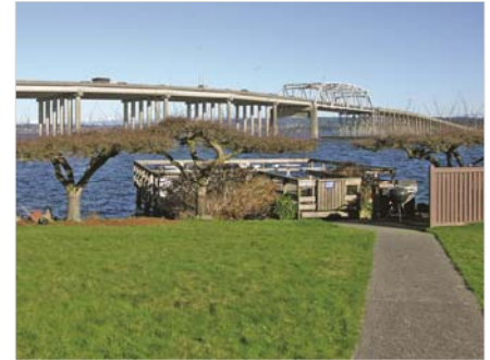
Bridge profile near Madison Park
