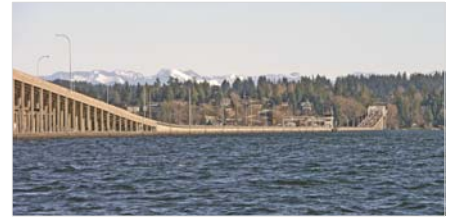
Evergreen Point Bridge (floating span in center)
