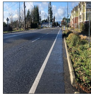
Suburban stormwater management buffer
