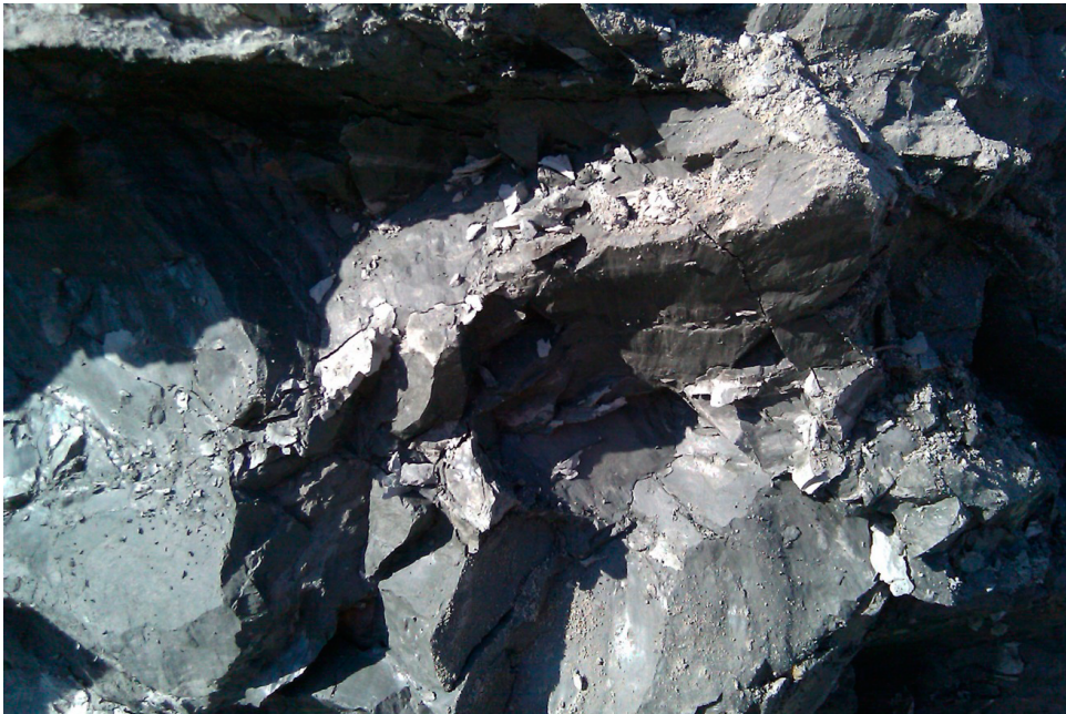
Exposure Near the East End of Sr-520 Illustrating Fractured and Sheared Structure Within Glacially Overridden Clay Deposit Believed to be Due to Glaciotectonics (a) Overview of Exposure, (b) Close-Up Showing Clay Structure Figure 5-2(b)
