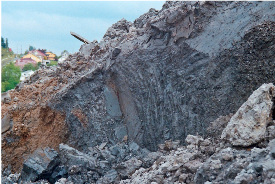
Example on Beacon Hill of Highly Disturbed Glacially Overconsolidated Clay Associated with a Paleolandslide Deposit; Note Near-Vertical Orientation of Laminae/Bedding Within the Landslide Block
