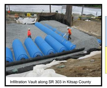
**Description:** Bottomless underground structures used for temporary storage and infiltration of stormwater runoff to groundwater. May be modified for runoff treatment.
