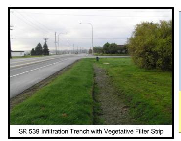
**Description:** Long, narrow, stone-filled trench used for collection, temporary storage, and infiltration of stormwater runoff to groundwater. Can be placed beneath parking areas, along site periphery, or other linear areas. Can be designed for runoff treatment.
