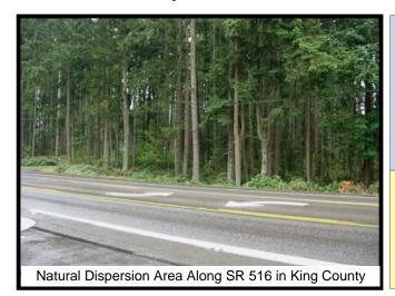
**Description:** Existing soils, vegetation, and topography are used to provide flow control and runoff treatment. Runoff enters the dispersion area as sheet flow and disperses into the surrounding landscape. It requires little or no construction activity.
