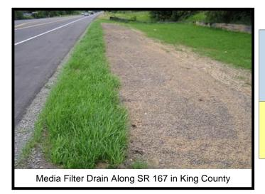
**Description:** Linear flow-through stormwater runoff treatment device along highway side slopes, medians, borrow ditches, and other linear depressions.
