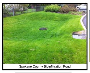
**Description:** Combines grasses or other vegetation and soils to remove stormwater pollutants by filtration, soil sorption, and uptake by vegetative root zones. Used in eastern Washington only.
