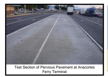
**Description:** The pervious concrete or asphalt pavement surface is an open-graded mix placed in a manner that results in a high degree of interstitial spaces or voids within the cemented aggregate. This technique allows runoff to infiltrate through to the subsoils.
