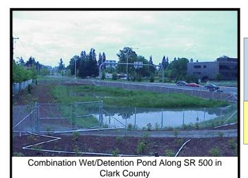
**Description:** Combination detention and runoff treatment wet pond. Looks like a detention facility, but has a permanent pool of water as well. Two sizes: basic and large.
