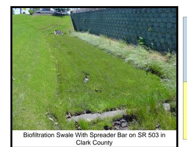
**Description:** Vegetation-lined channels designed to remove suspended solids from stormwater. Shallow concentrated flow, allows for the filtration of stormwater by soil, plants, and leaves.
