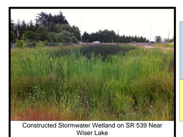
**Description:** Shallow constructed wetlands. Designed to treat stormwater through settling, filtering, and biological processes associated with aquatic plants. Over time, pollutants concentrate in the sediment.
