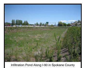
**Description:** Used for collection, temporary storage, and infiltration of stormwater runoff to groundwater. For flow control and can be designed to provide runoff treatment.
