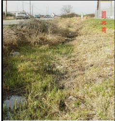
Wet Biofiltration Swale along I-5 in Snohomish County **Description:** Variation of basic biofiltration swale. Vegetation is specifically selected for areas where water tables are high, or continuous base flow results in saturated soil conditions.
