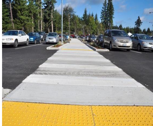
Pedestrian Access Route
