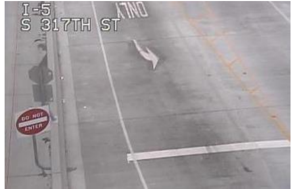
Do Not Enter sign located on the left side at the top of each off-ramp.
