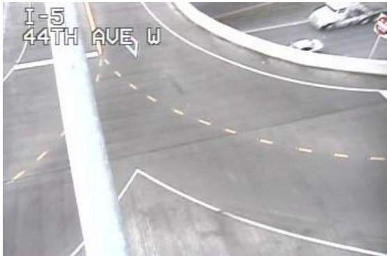
Guide striping provided for left-hand turns.
